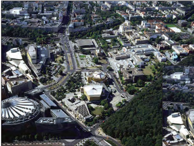
Aerial photo (view from north)
